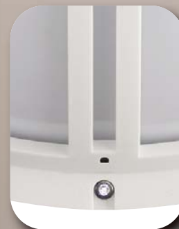
Tamperproof screws and drain hole
